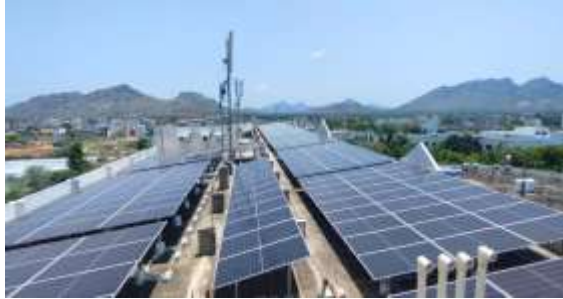
250 kW rooftop solar PV system on Saraswathi Block.
